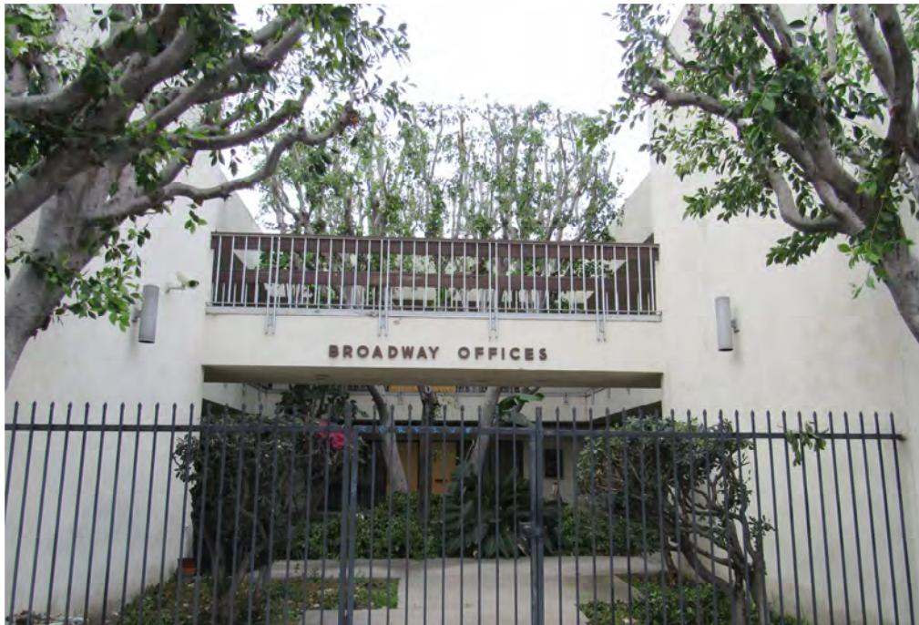
Photograph 1. View of office complex located south of Broadway.
