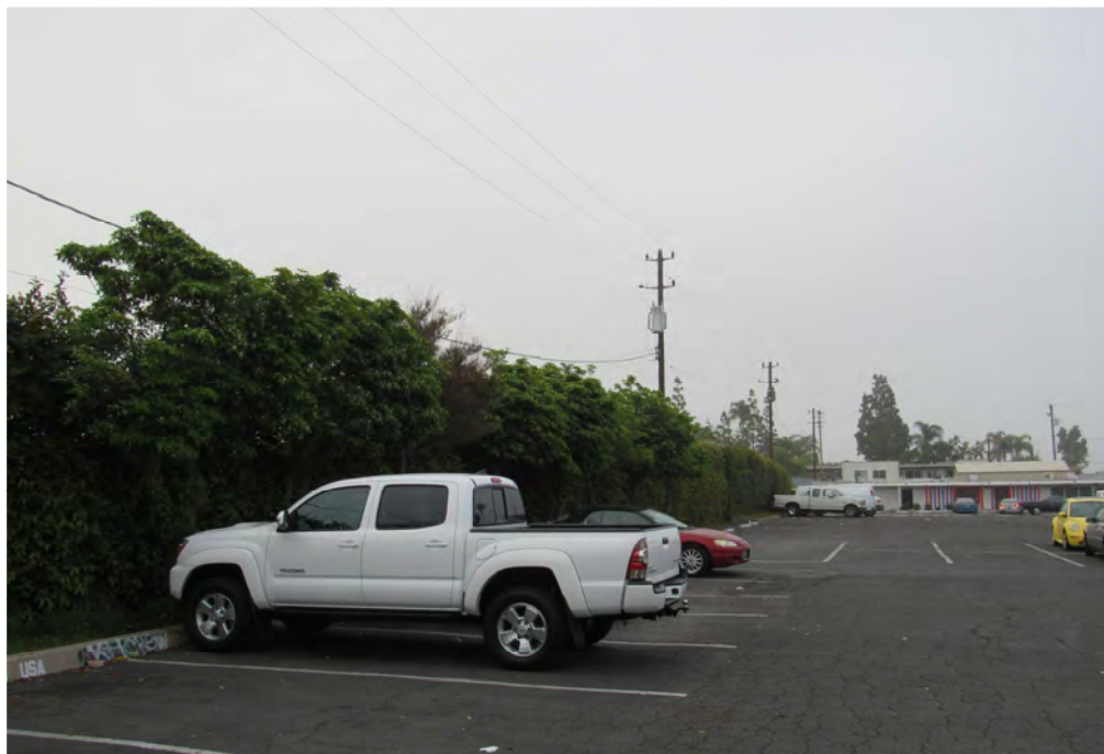
Photograph 2. View looking south of the vegetated block wall located along the eastern property boundary.
