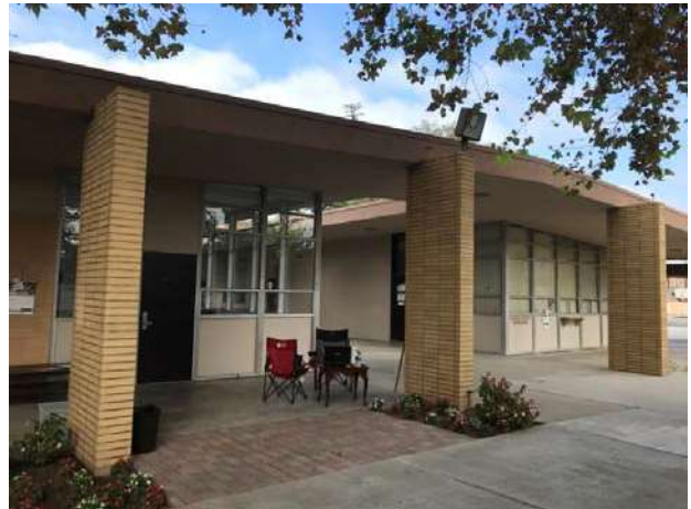
6. Additional view of the Main Office Building.
