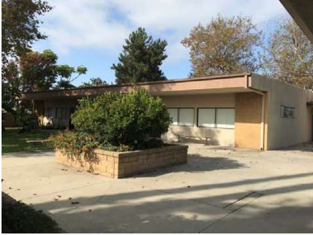
7. View of the a classroom building.
