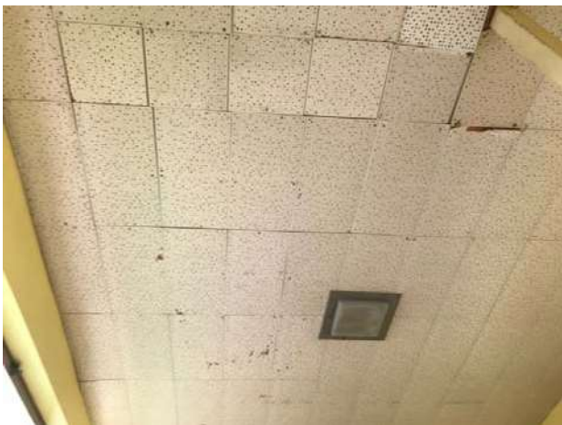
39. View of ceiling tiles.
