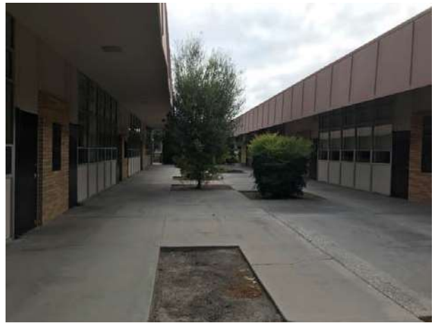
4. View of the classroom building within the southeastern corner of the parcel
