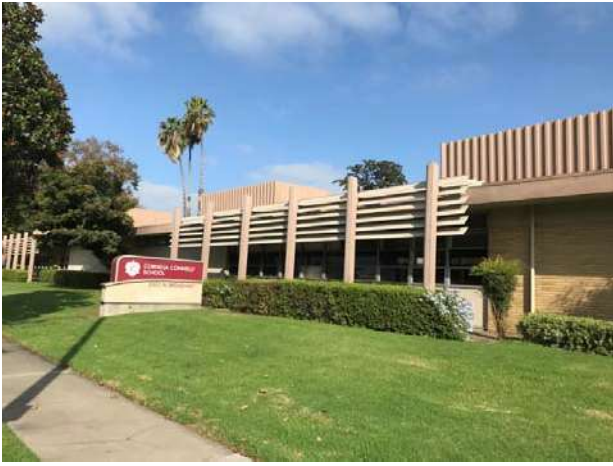
1. View of the subject property facing northwest along West Broadway.
