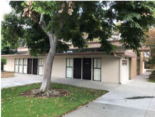
5. View of the Main Office Building.
