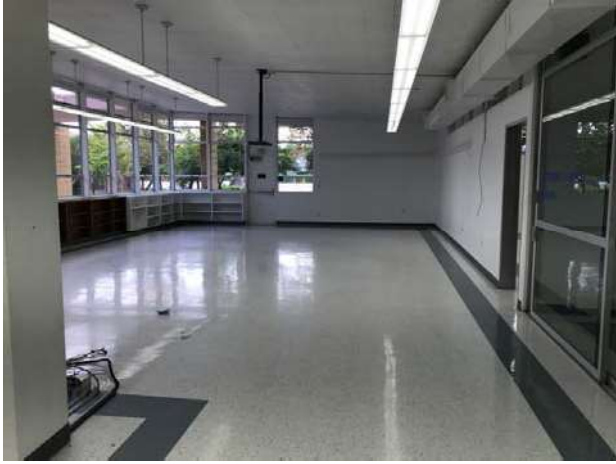
25. View of the main office space.
