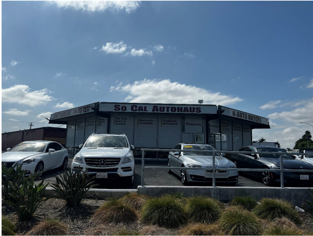
Photo 1: Overview of structure 1200 S Anaheim Blvd. View S.
