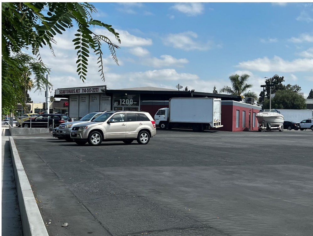
Photo 2: Overview of structure 1200 S Anaheim Blvd. View NE.
