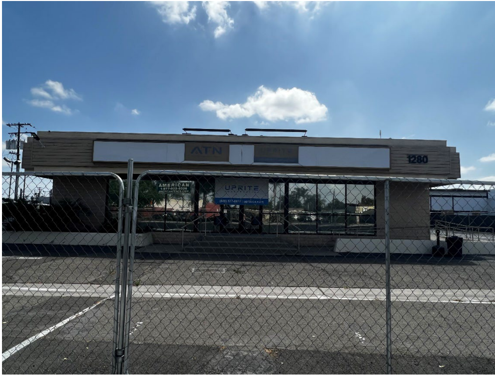
Photo 7: View of 1280 S Anaheim Blvd. View E.
