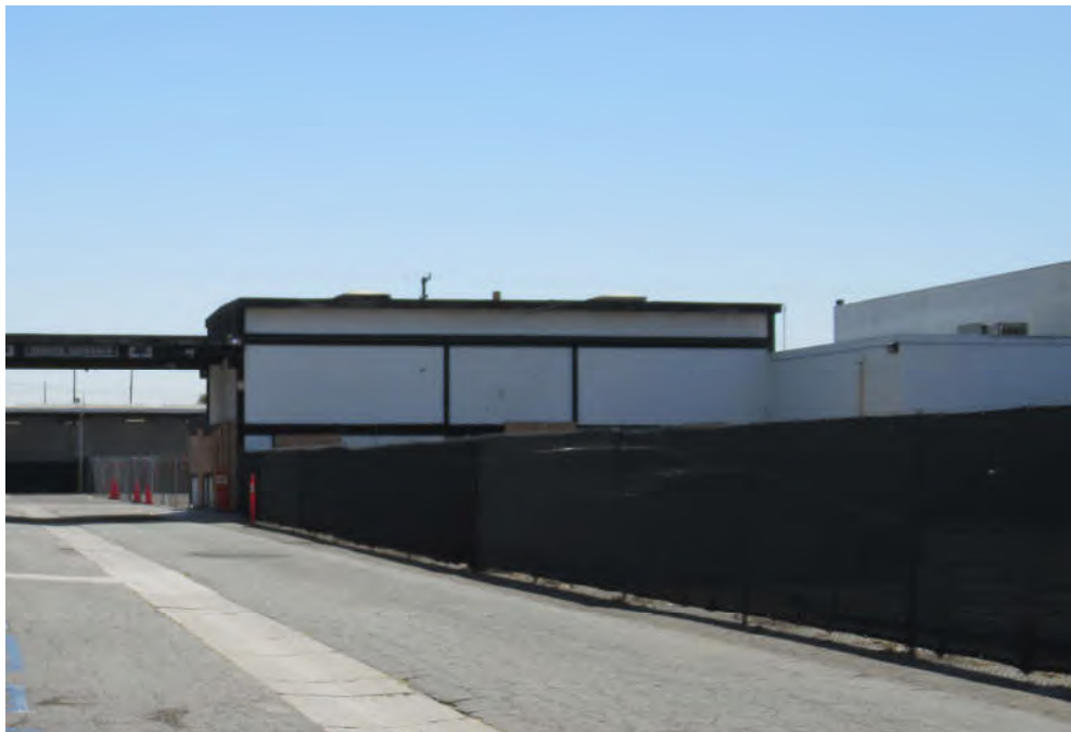
Photograph 2. Ancillary building, west elevation, view east
