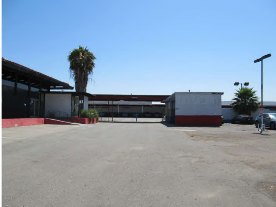
Photograph 3. Service building, view east.
