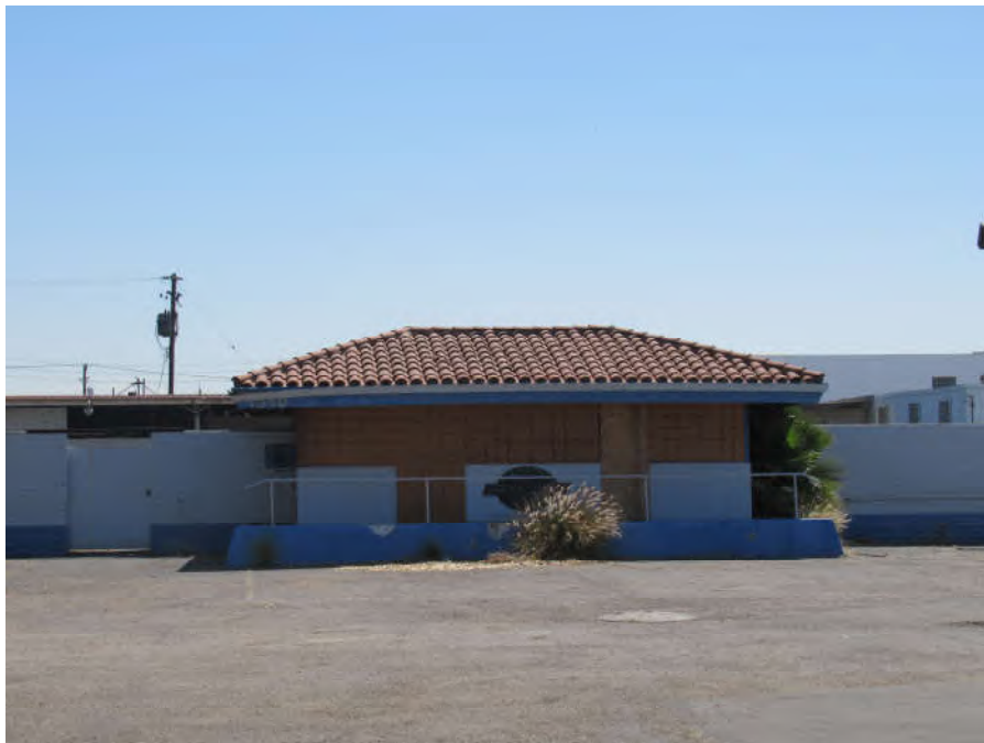
Photograph 4. Ancillary building, west elevation, view east.
