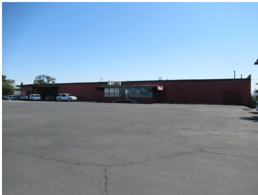
Photograph 4. Service building, west wing, view east.
