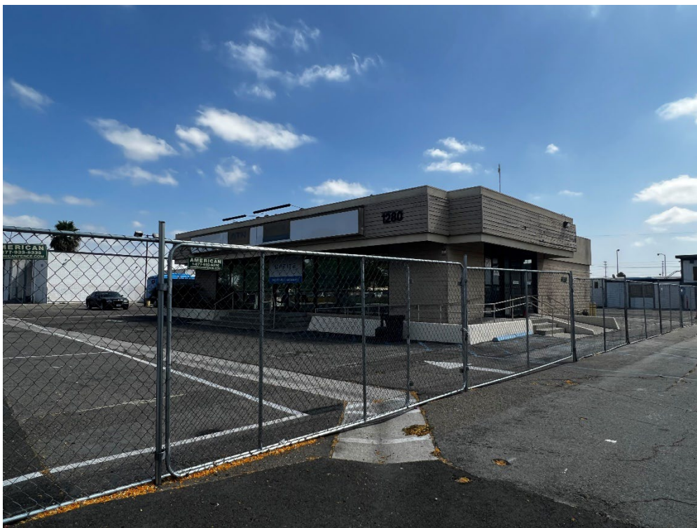
Photo 8: View of 1280 S Anaheim Blvd. View NE.
