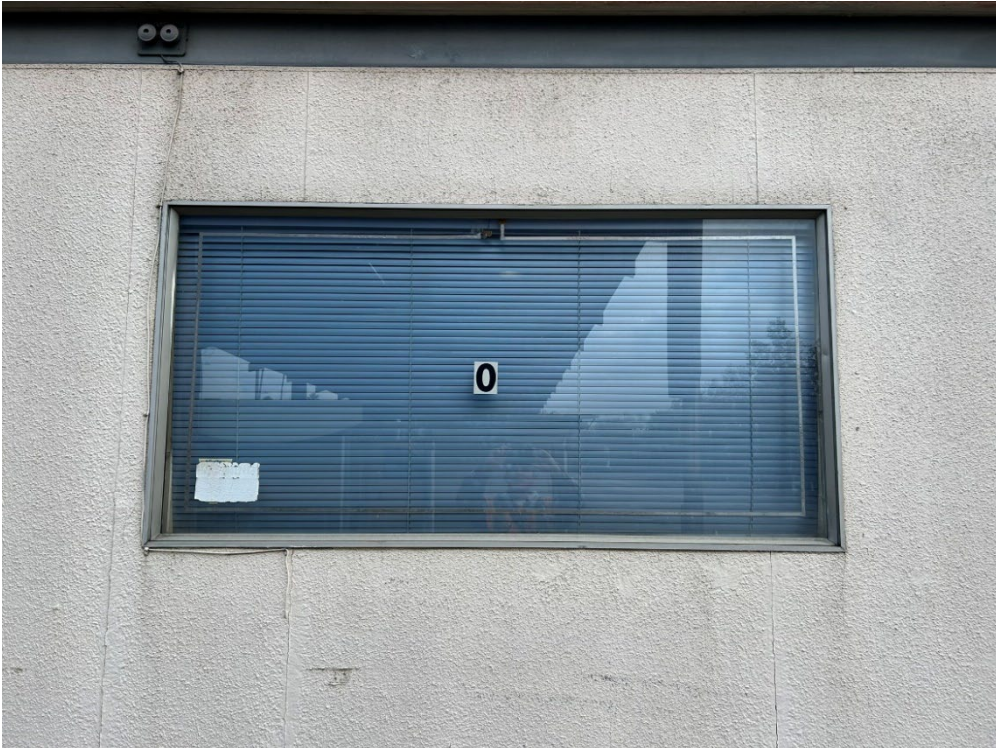
Photograph 27: View of aluminum single pane window on west elevation, facing east.
