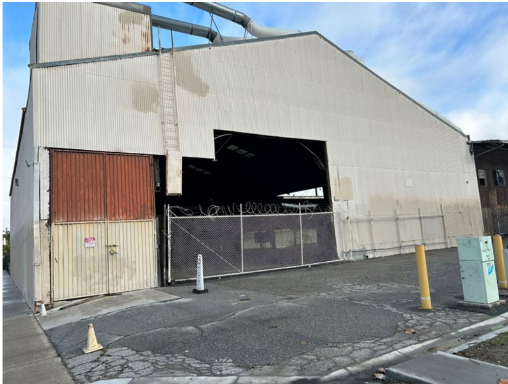
Photograph 54: Overview of southwest corner of structure, looking northeast.
