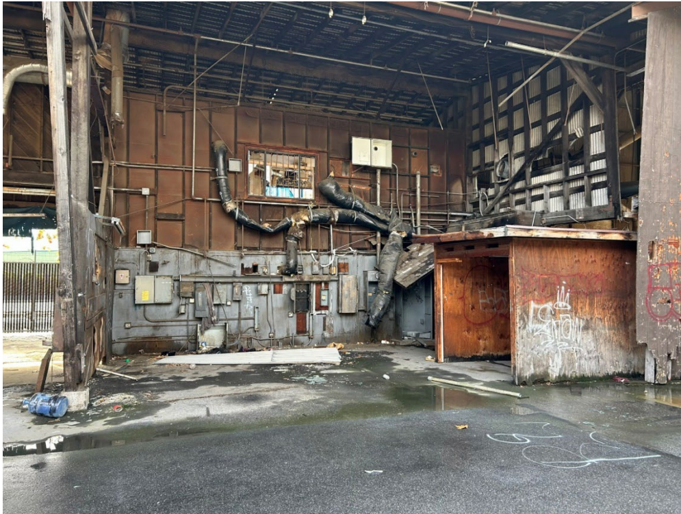
Photograph 43: Overview of interior of structure, facing south.
