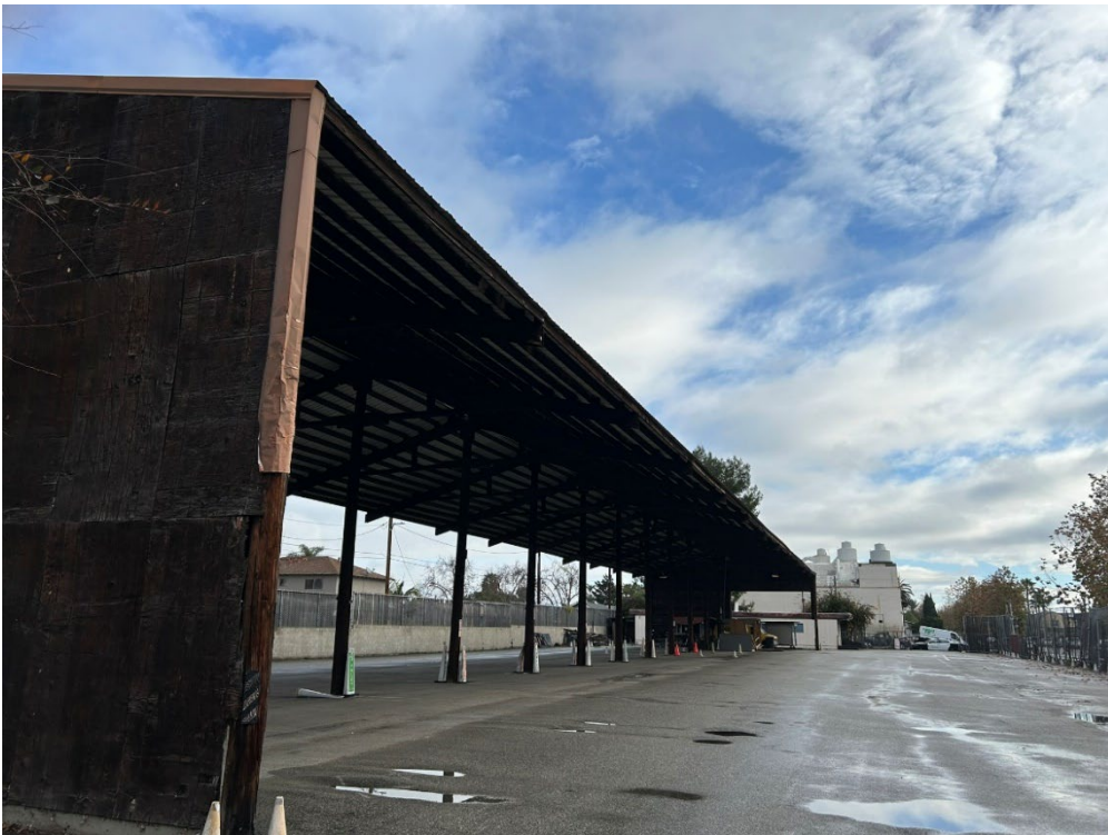
Photograph 12: View of south elevation of shed from southwest corner, facing northeast.
