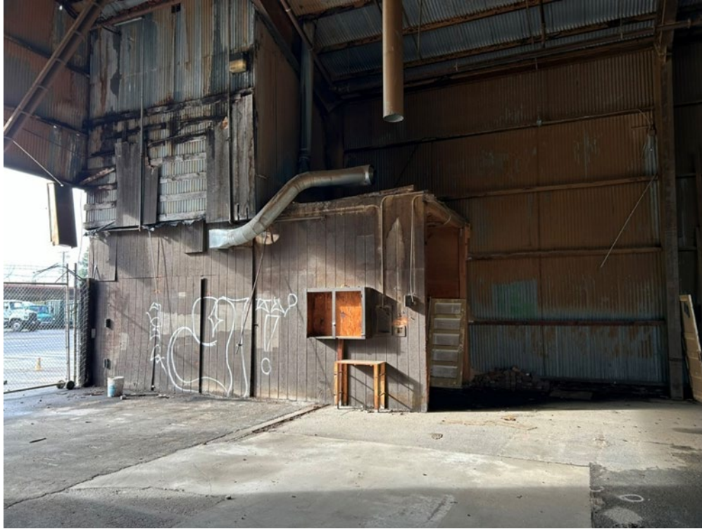
Photograph 41: View of interior of structure, facing southwest.
