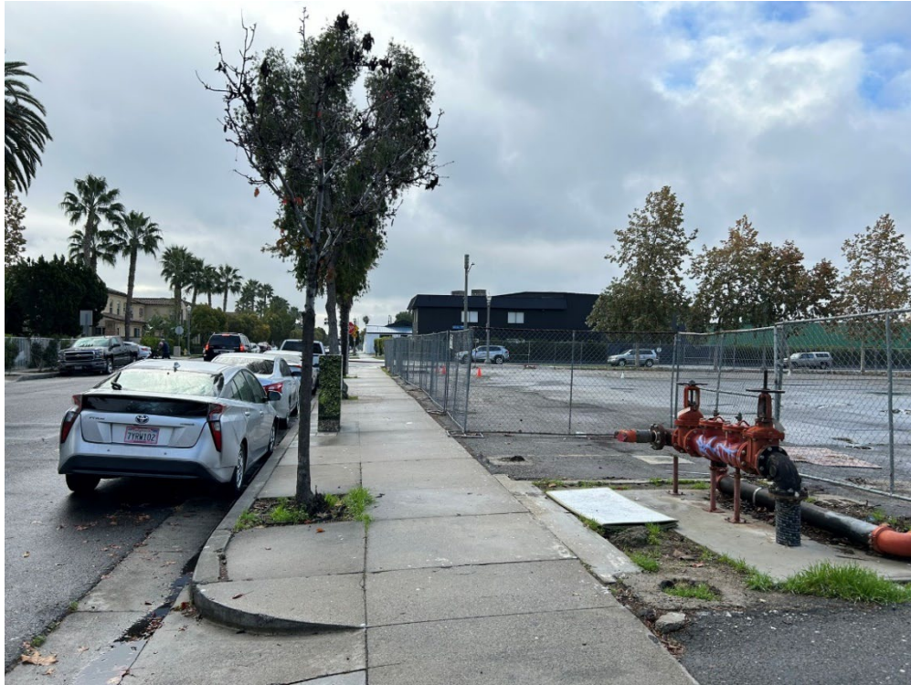
Photograph 33: Overview from Olive Street, and unnamed alley, facing south.
