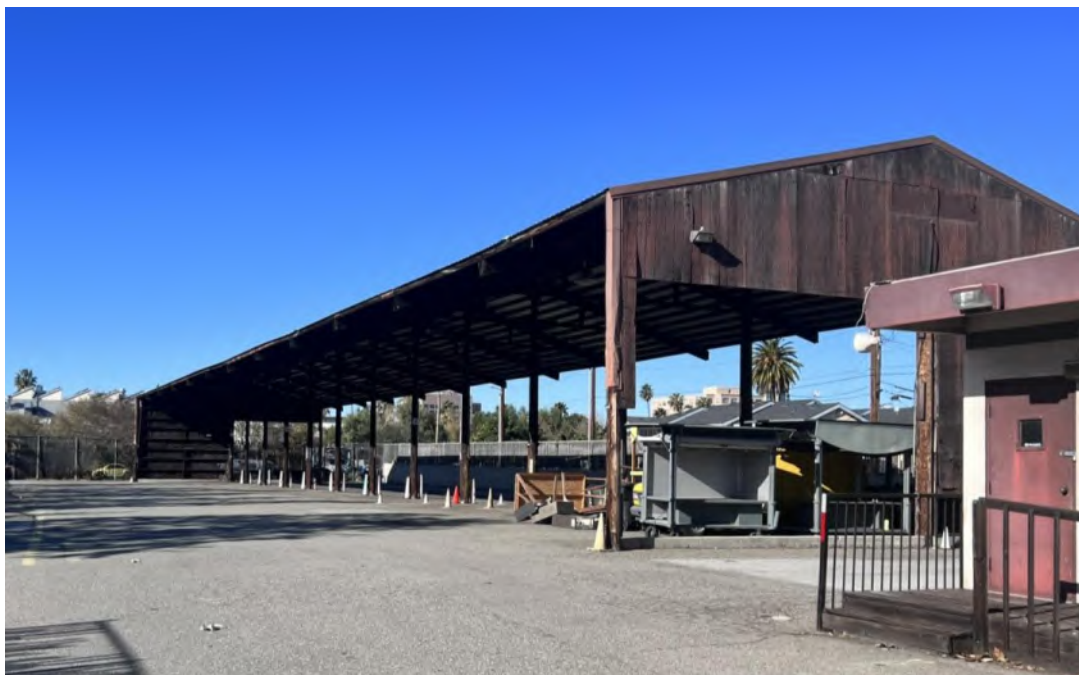
Photograph 7. Building 2, view northwest
