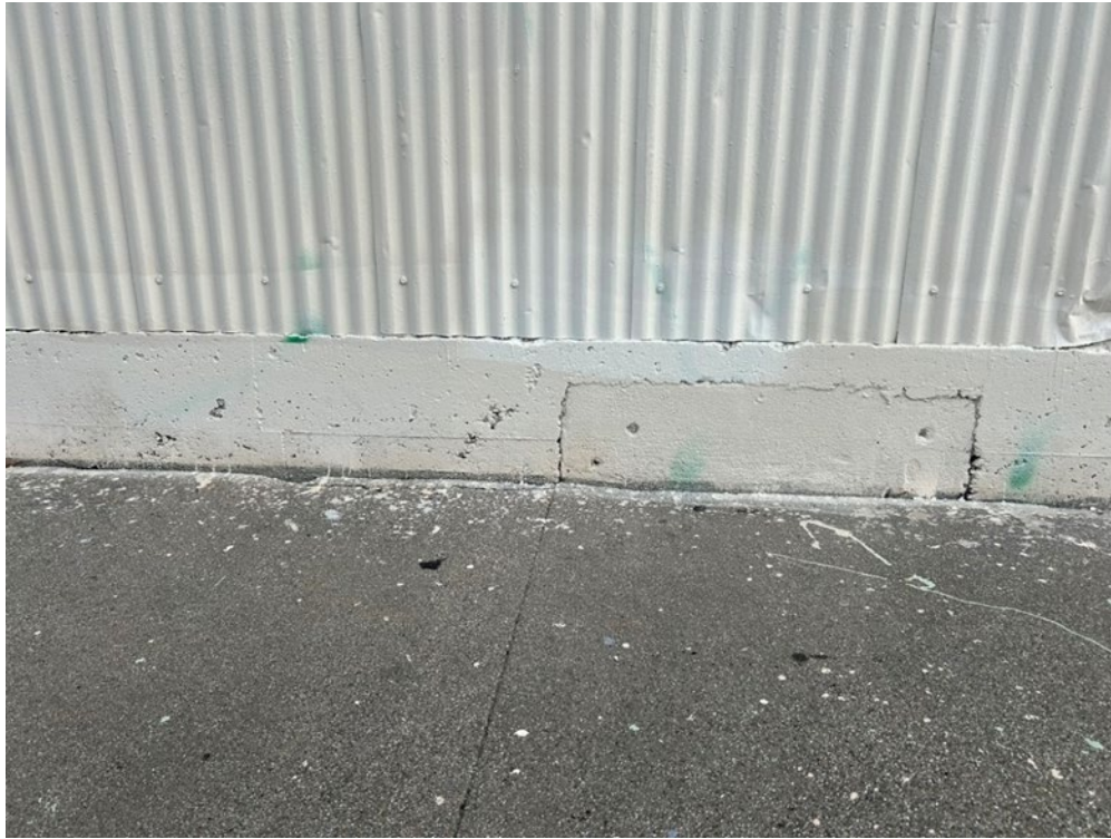
Photograph 53: Overview of foundation at west elevation, facing east.
