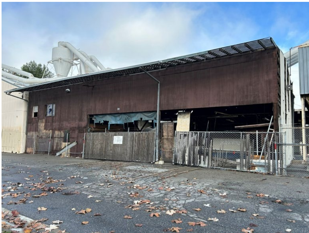
Photograph 58: Overview near center of south elevation, facing northwest.
