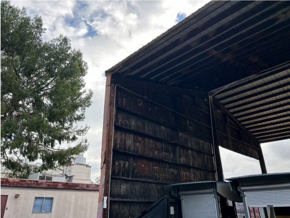
Photograph 15: View of northeast corner of shed, facing southeast.
