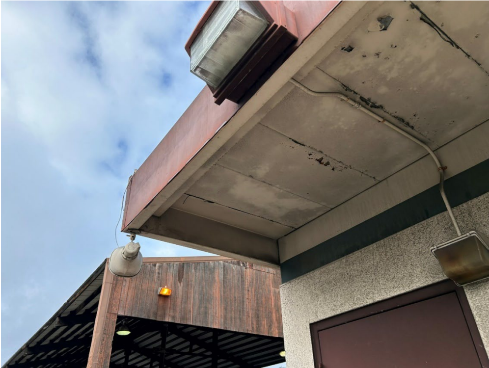
Photograph 19: View of eaves at southwest corner of building.
