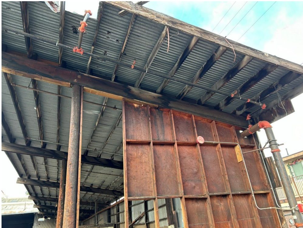
Photograph 37: View of eaves on structure at east end.
