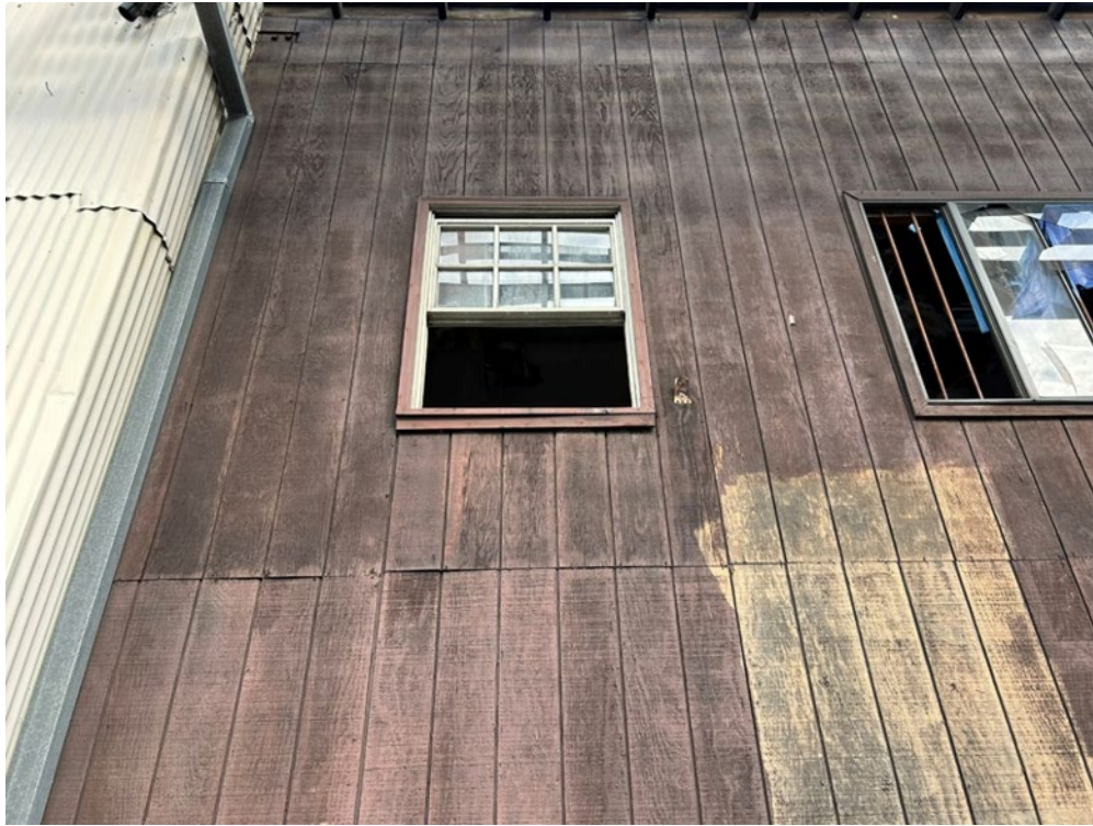
Photograph 49: View of aluminum paned window, facing north.
