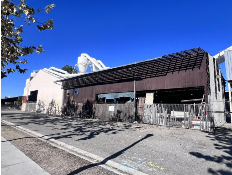
Photograph 3, Circa 1956 section of the building, south elevation, view northwest
