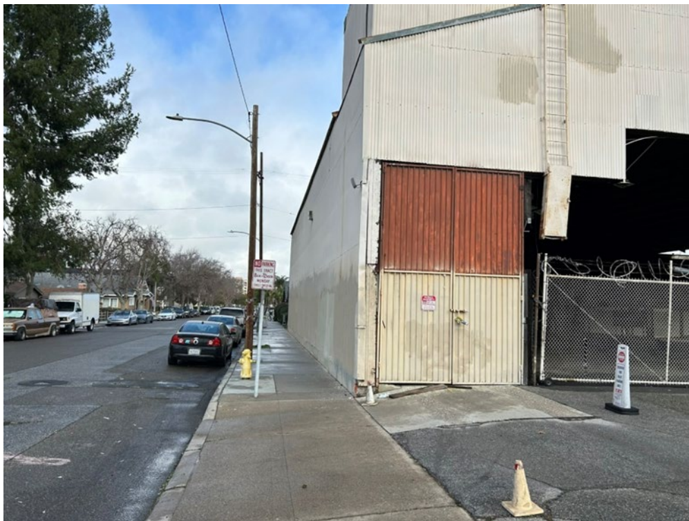
Photograph 50: Overview of southwest corner of structure near Philadelphia St, and Santa Ana Street, facing north.
