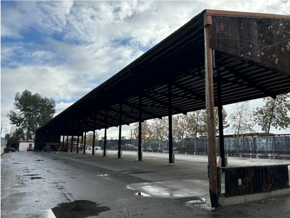
Photograph 11: View of north elevation of shed from northwest corner, facing southeast.
