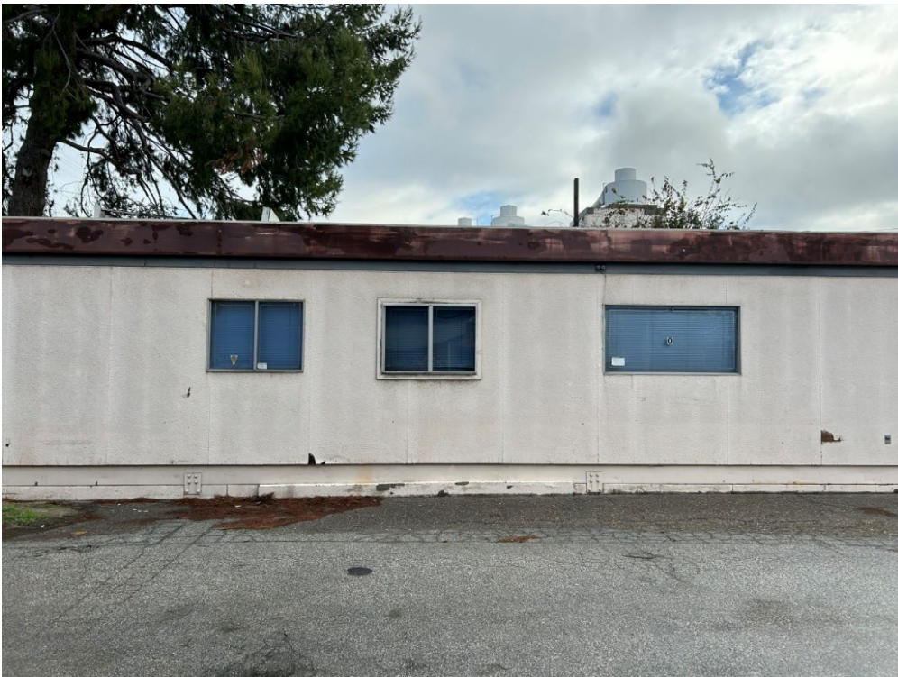
Photograph 20: View of west elevation of building, facing east.
