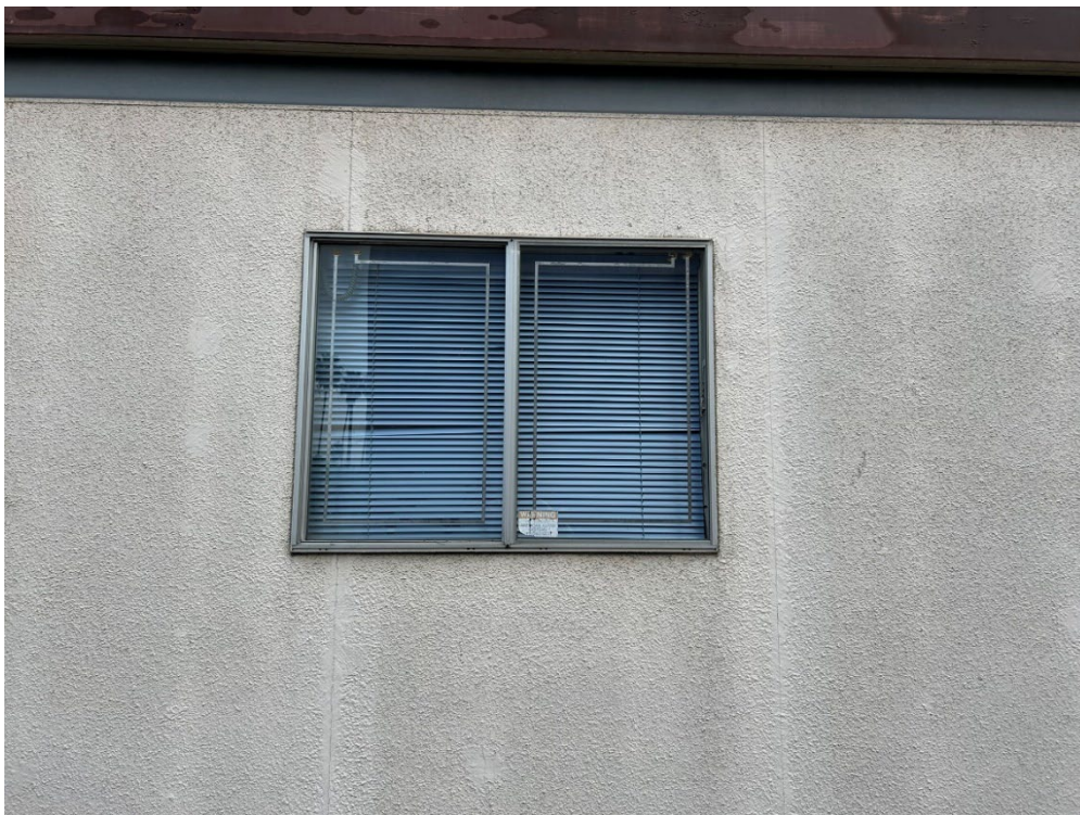
Photograph 24: View of aluminum, double pane window on west elevation, facing east.
