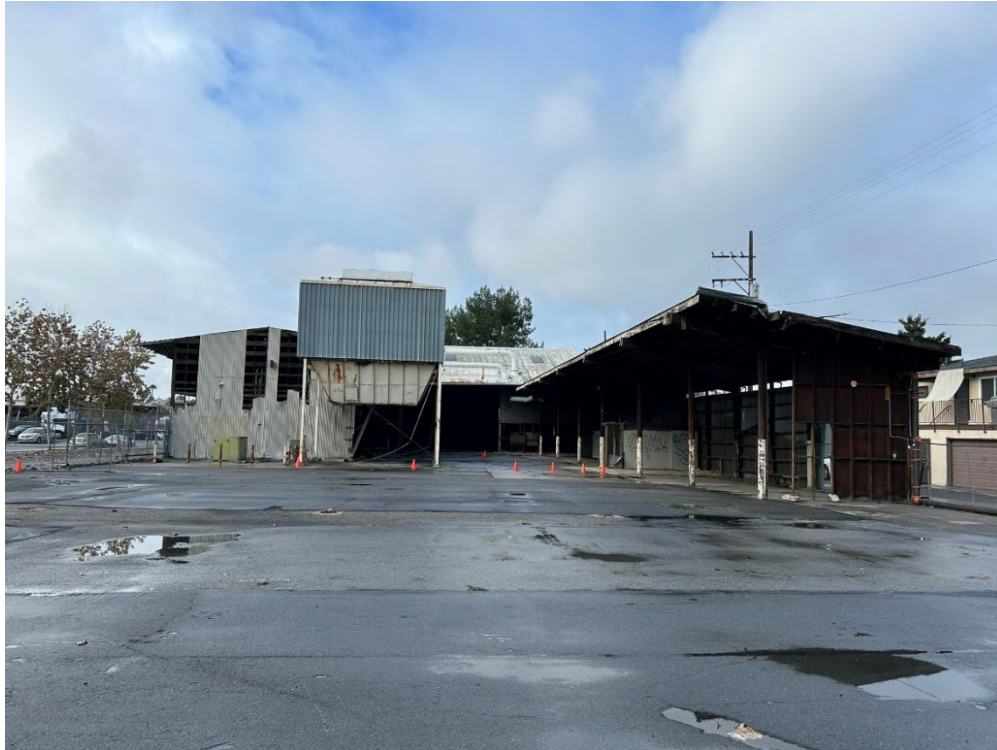
Photograph 37: Overview of east elevation of structure, facing west.
