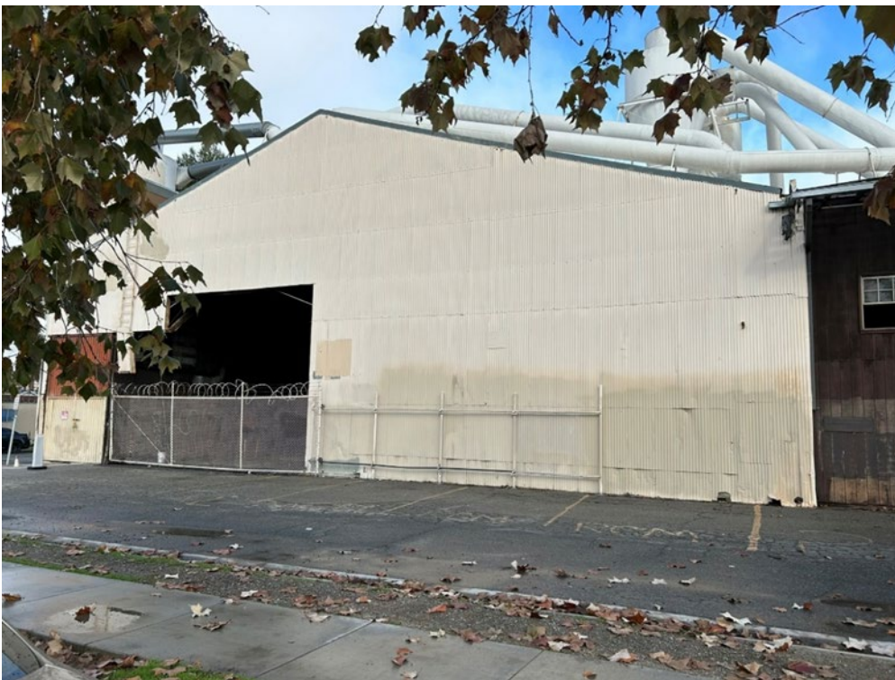
Photograph 56: Overview southwest portion of structure, facing northwest.
