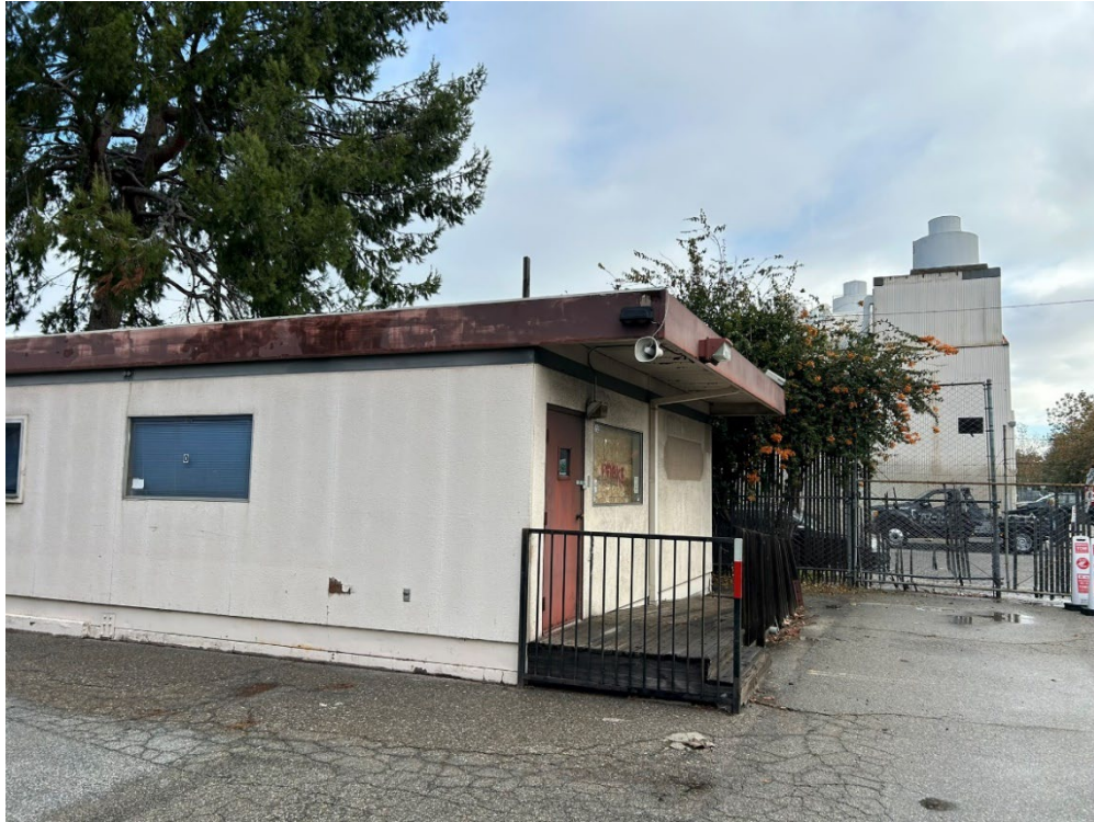
Photograph 21: View of southwest corner of building, facing northeast.
