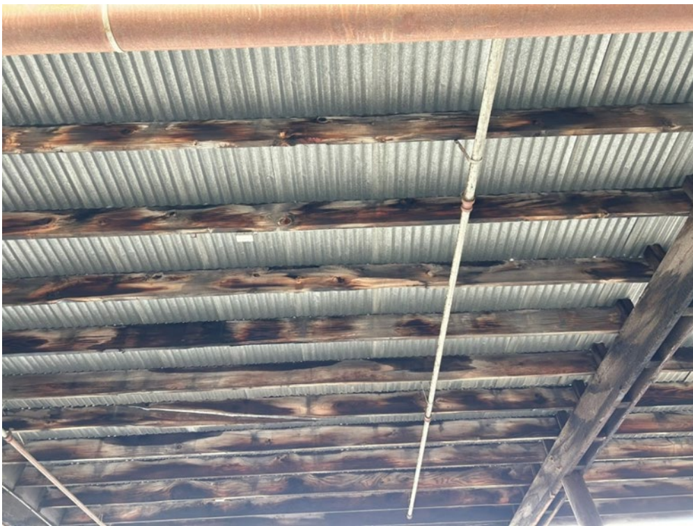
Photograph 62: View of interior ceiling of structure.
