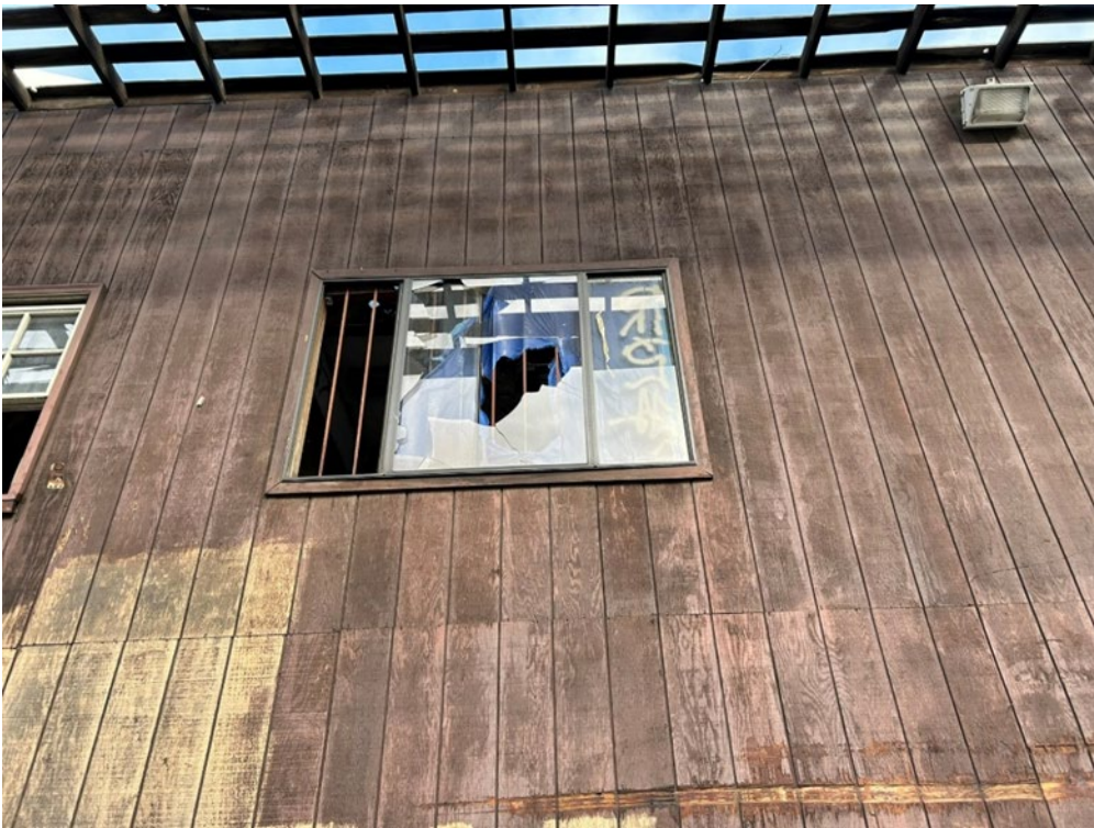
Photograph 48: View of aluminum framed sliding glass window, facing north.
