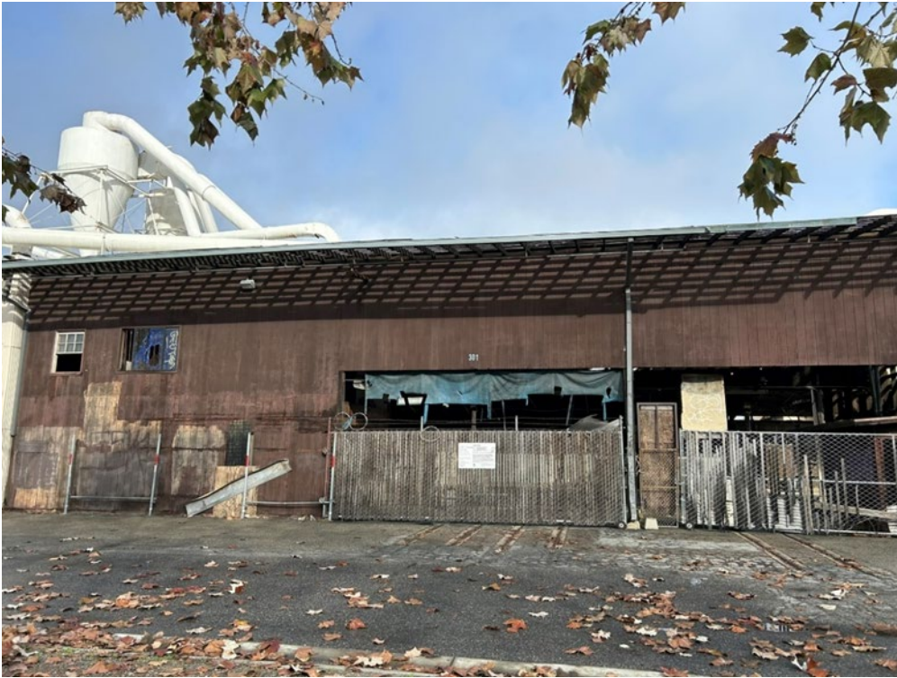
Photograph 47: Overview of south elevation near center of structure, facing north.
