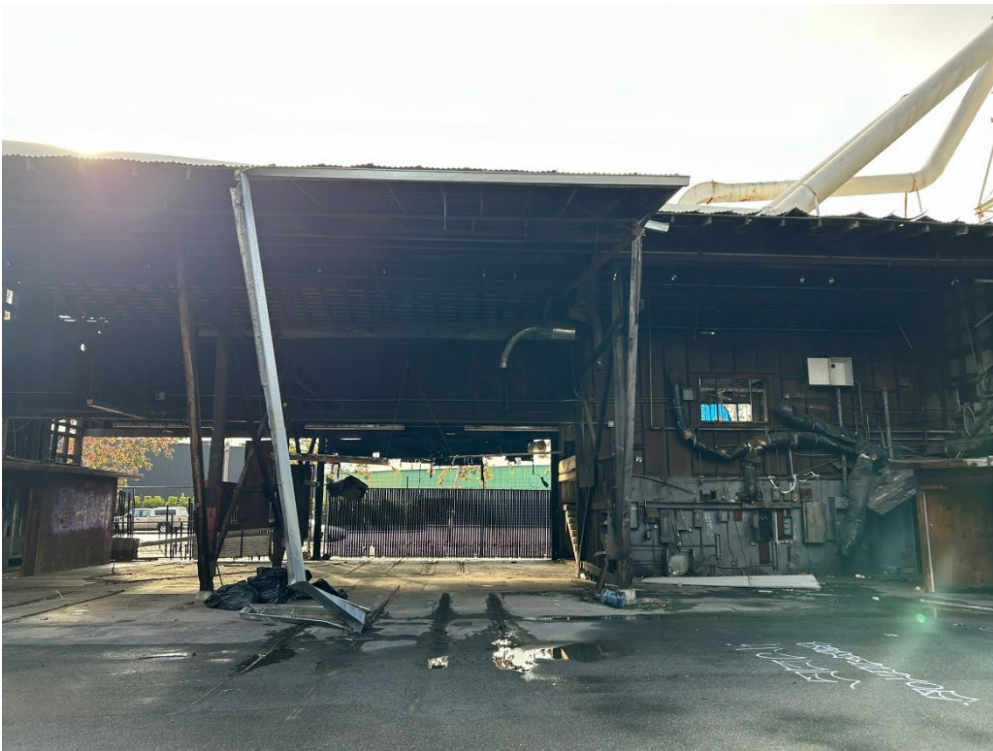
Photograph 40: Overview center of structure, facing south.
