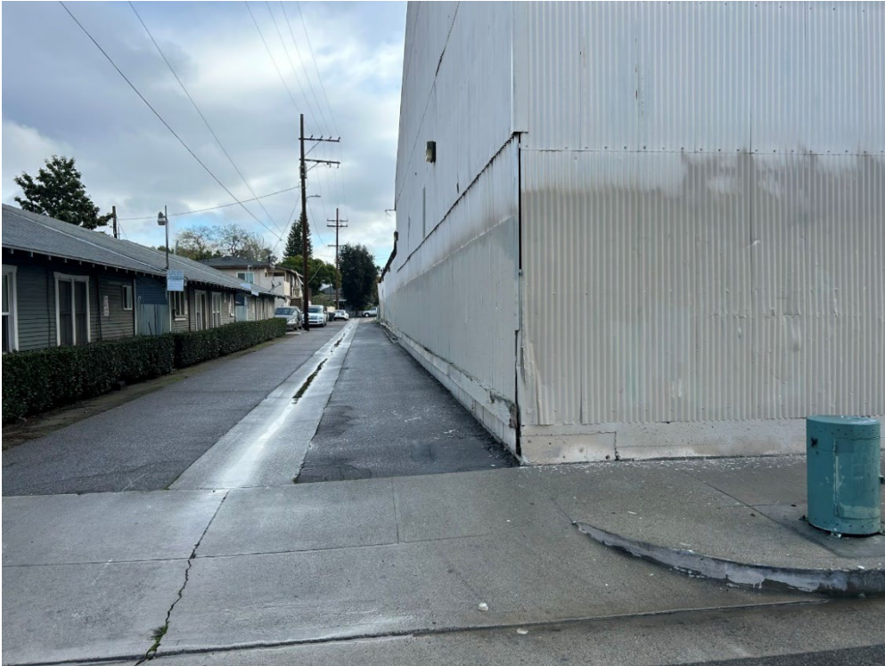
Photograph 35: View of northwest corner of structure at 301 E. Santa Ana Street, facing east.
