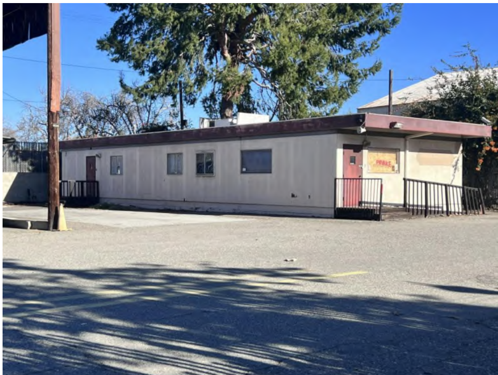
Photograph 8. Building 3, west and south elevations, view northeast
