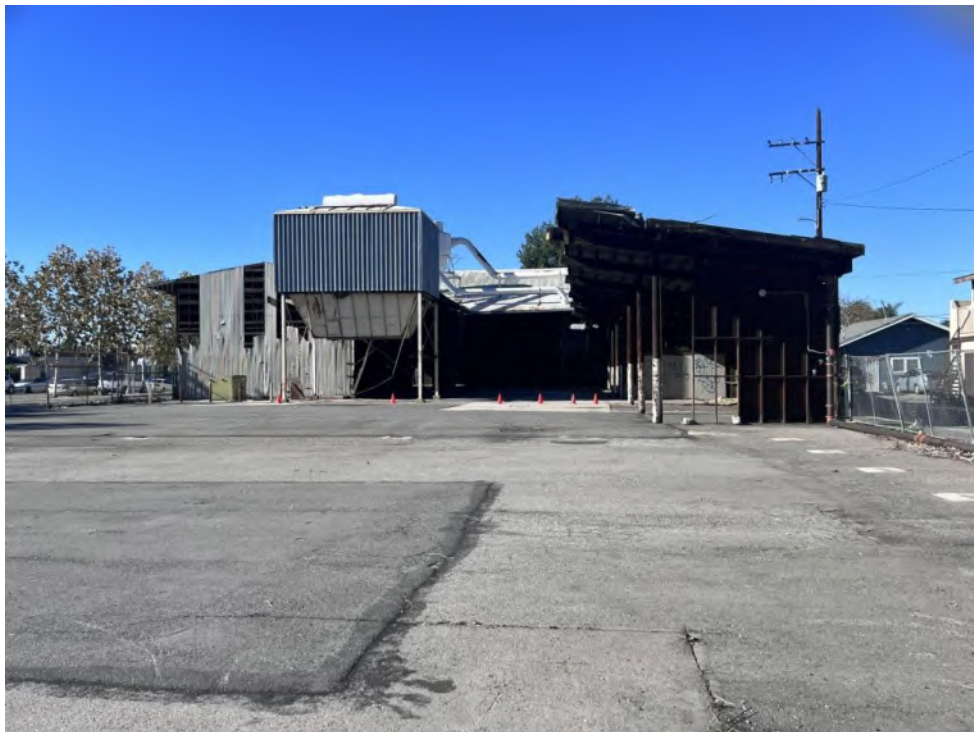
Photograph 2. Building 1, east elevation, view west
