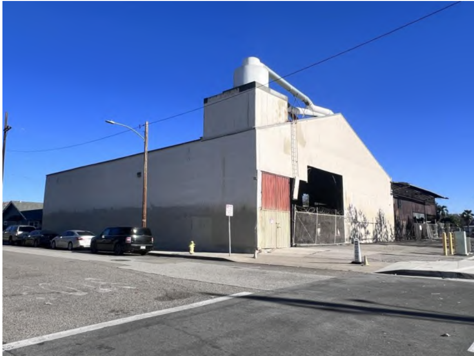
Photograph 5. Building 1, 1959 section of the building, west and south elevations, view northeast
