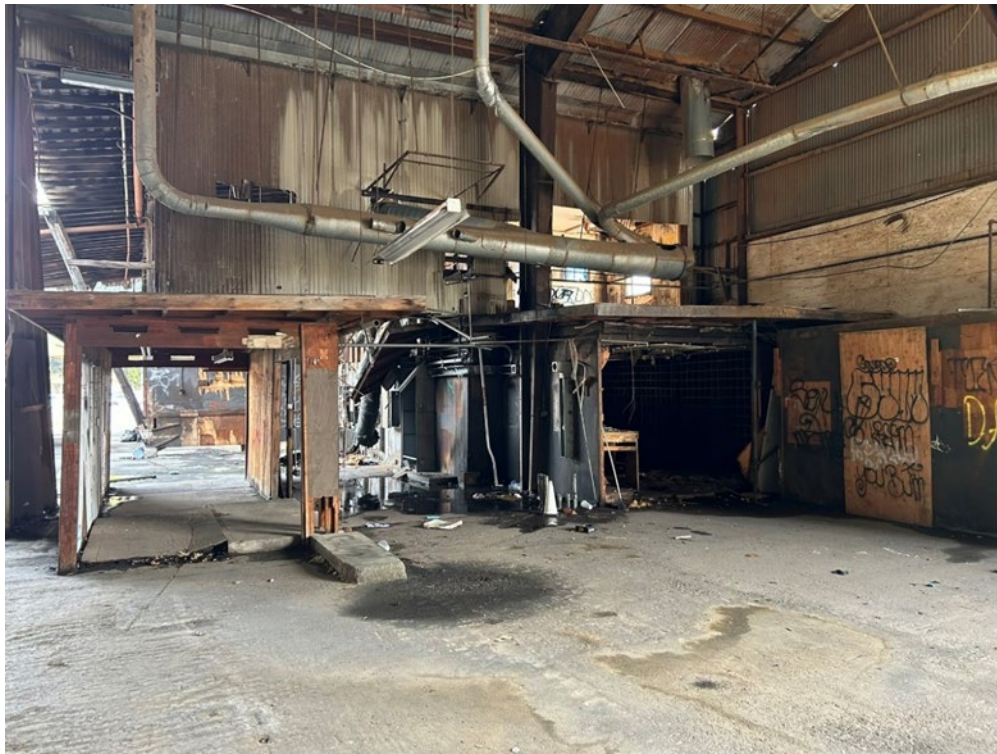
Photograph 42: View of interior of structure, facing southeast.
