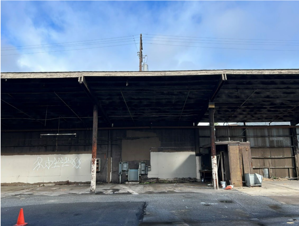
Photograph 39: Overview of center of structure, facing north.
