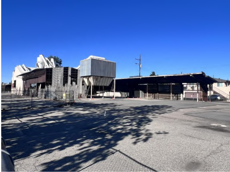
Photograph 1 Building 1 south and east elevations, view northwest
