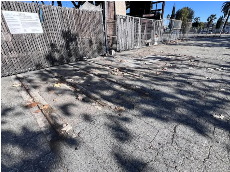
Photograph 4. Railroad spurs leading into Building 1, view northeast
