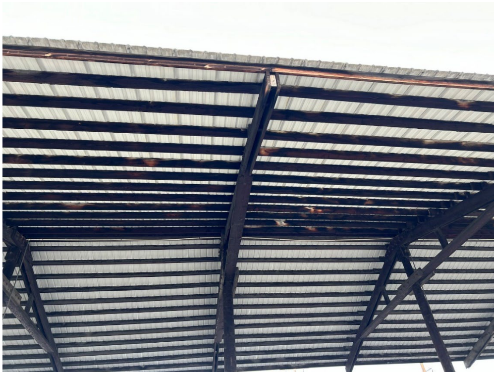
Photograph 14: View of truss, supports, and ceiling.
