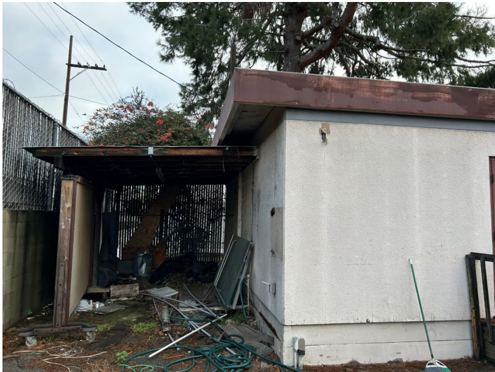
Photograph 22: View of northwest corner of building, facing southeast.
