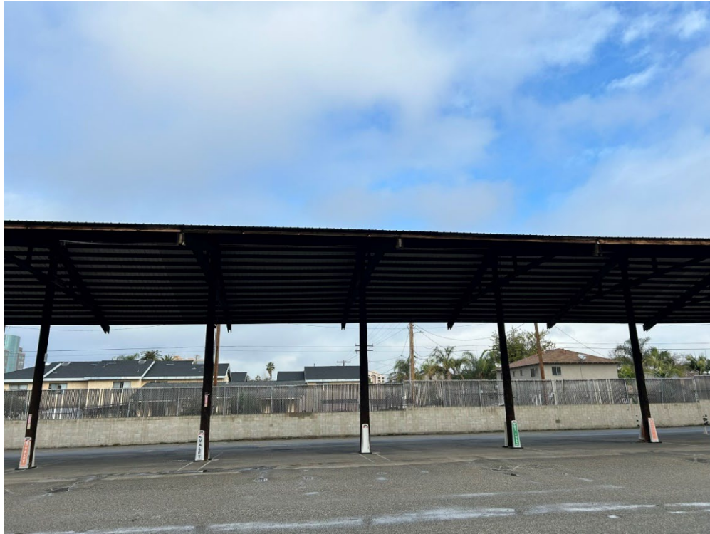
Photograph 13: View of south elevation from near center of shed, looking north.
