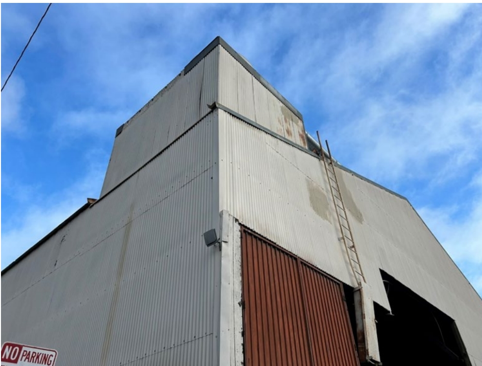
Photograph 52: Overview of southwest corner of structure, facing northeast.
