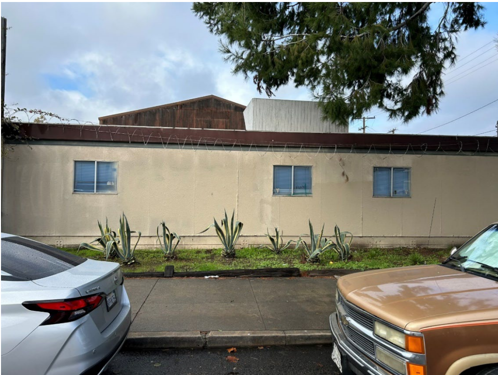
Photograph 28: Overview of east elevation of building and windows, facing west.
