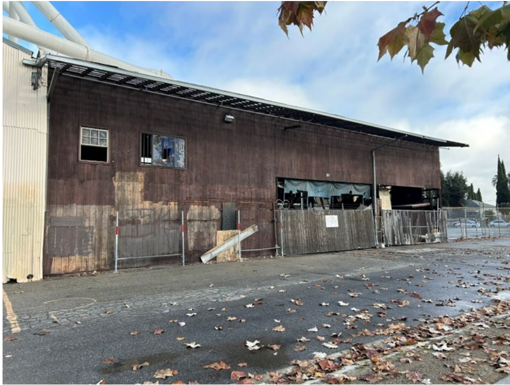
Photograph 57: Overview near center of south elevation, facing northeast.
