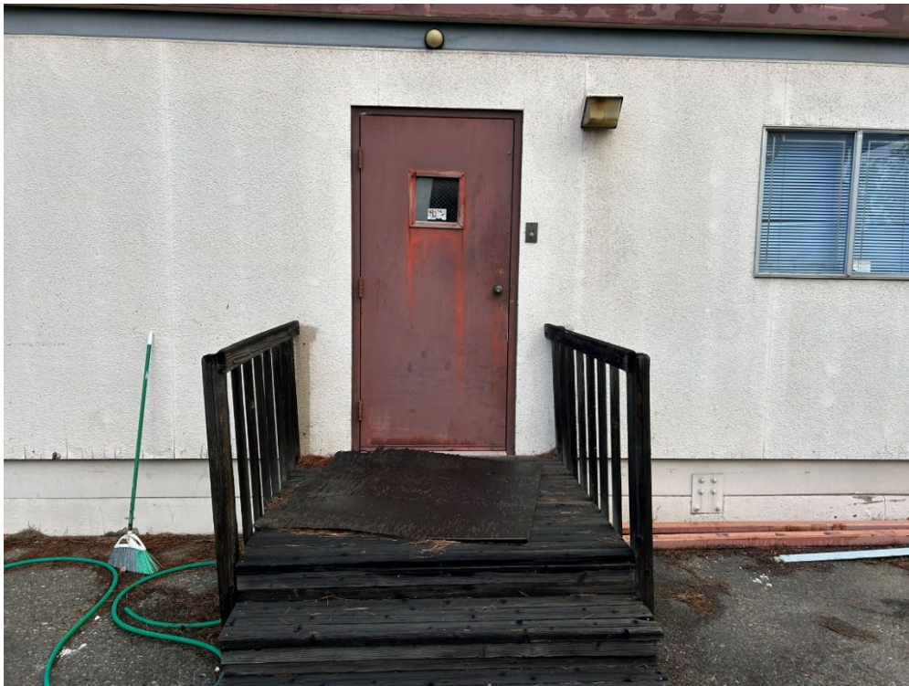
Photograph 23: View of redwood steps, landing, and steel door on west elevation of building, facing east.
