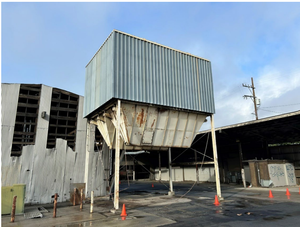
Photograph 44: Overview of "hopper" feature at east elevation of structure, facing northwest.
