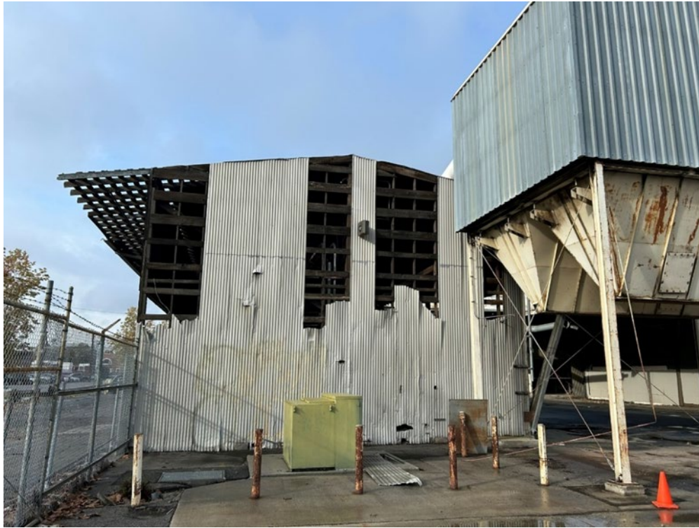
Photograph 45: Overview of east elevation of structure and hopper, facing west.
