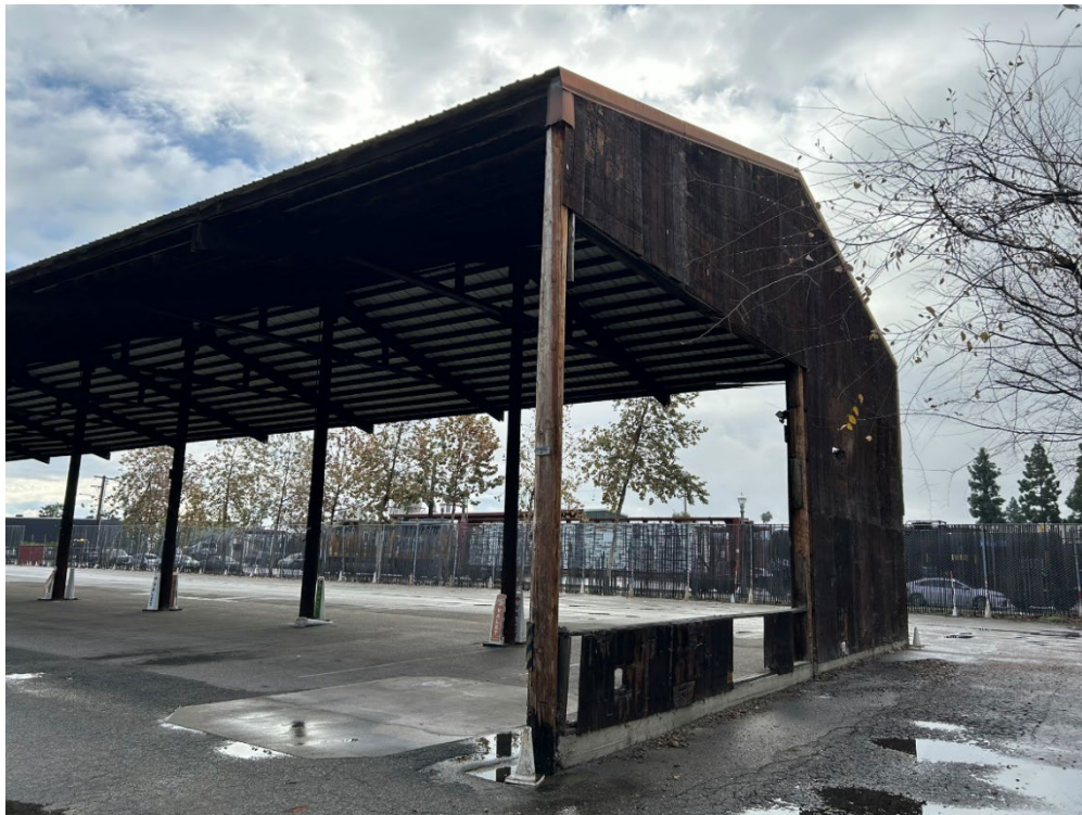
Photograph 10: View of northwest corner of shed, facing southeast.
