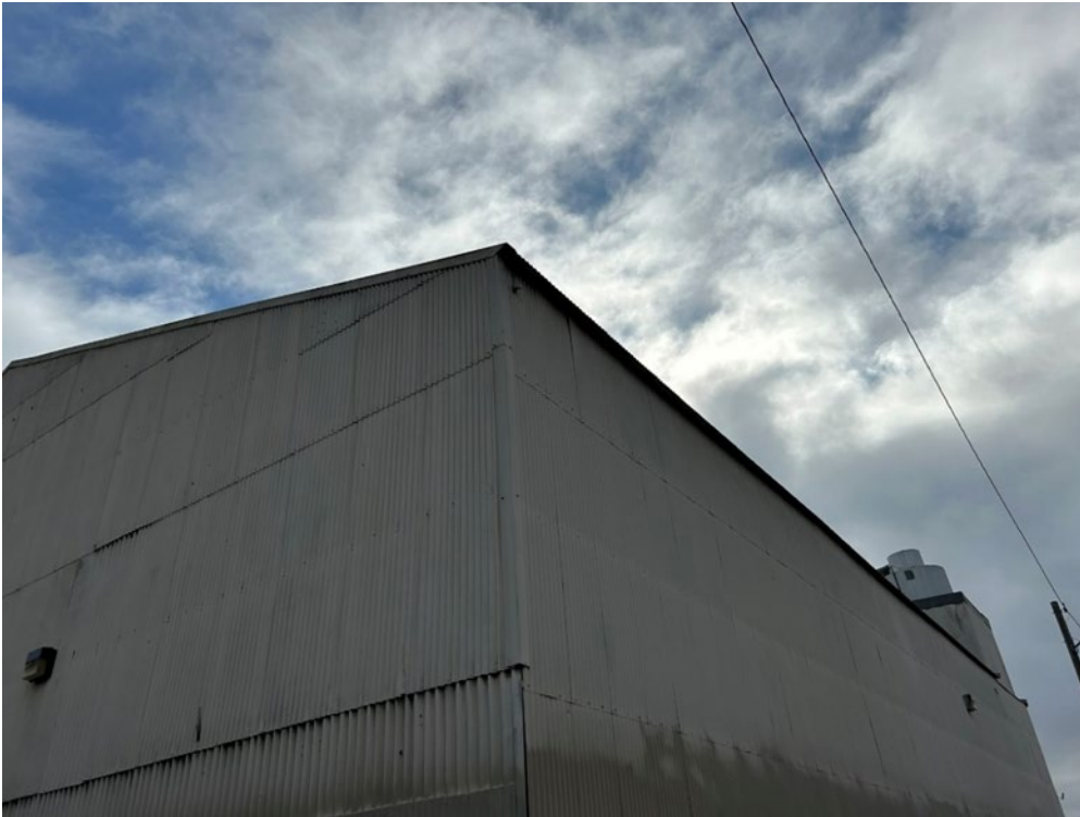
Photograph 59: Overview of northwest corner of structure, facing southeast.
