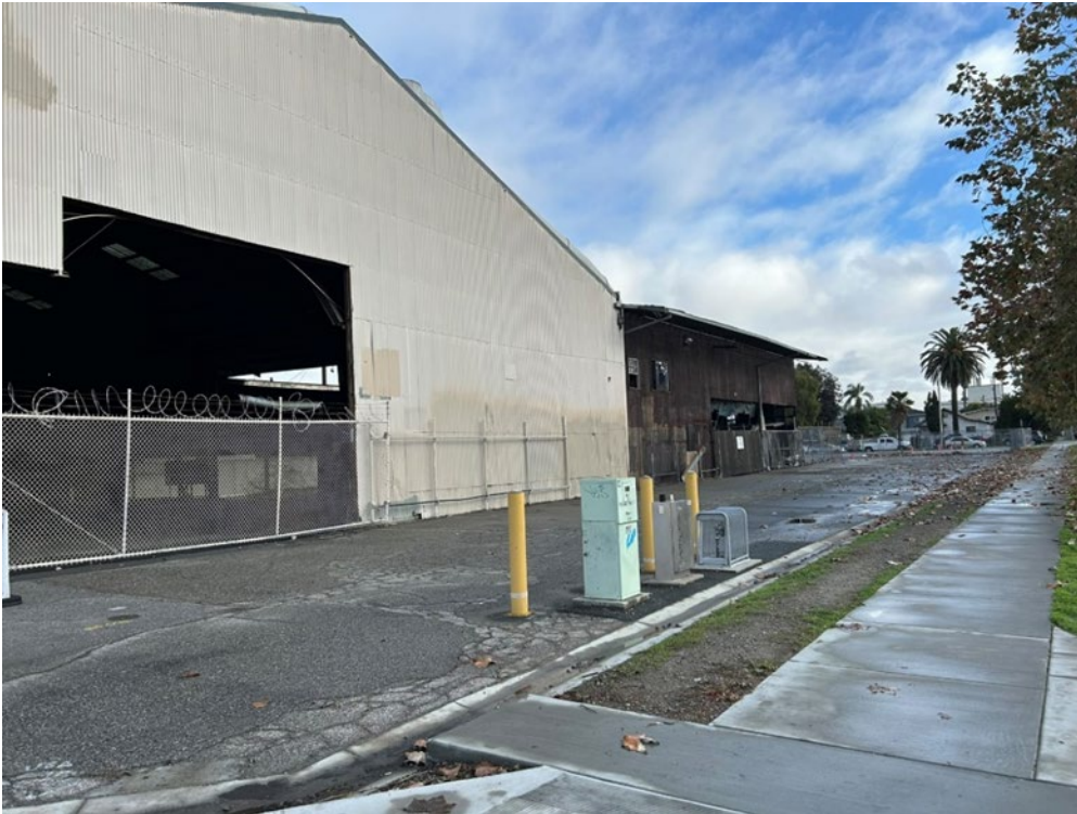
Photograph 55: Overview of south elevation, facing northeast.
