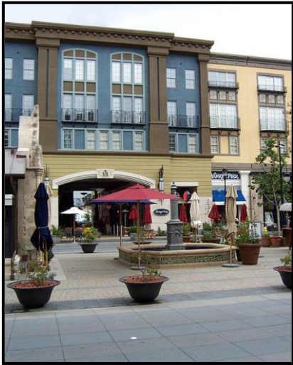
Detailed facade treatment – differing window styles, bays, and piers – reduces the scale of large, commercial buildings.
