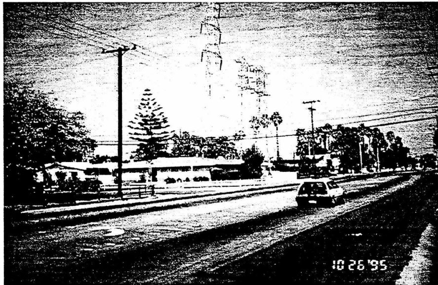
Existing SCE 66 kV/220 kV Transmission Lines - Crossing Walnut Street (Looking North)
