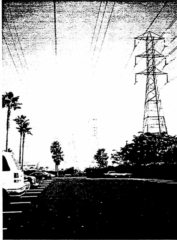
Existing SCE 66 kV/220 kV Transmission Lines - Across Disneyland Parking Lot (Looking East)
