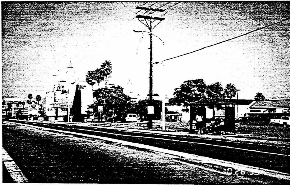
Harbor Boulevard - East Side (Looking North)
