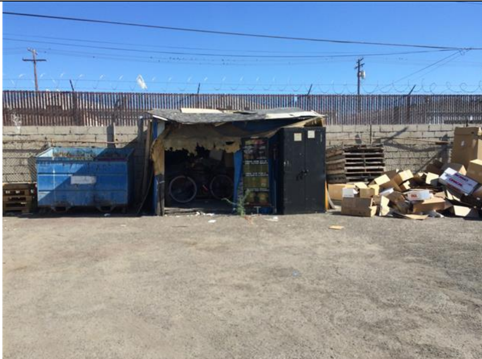
Photo #5 View of storage shed. No hazardous materials storage.
