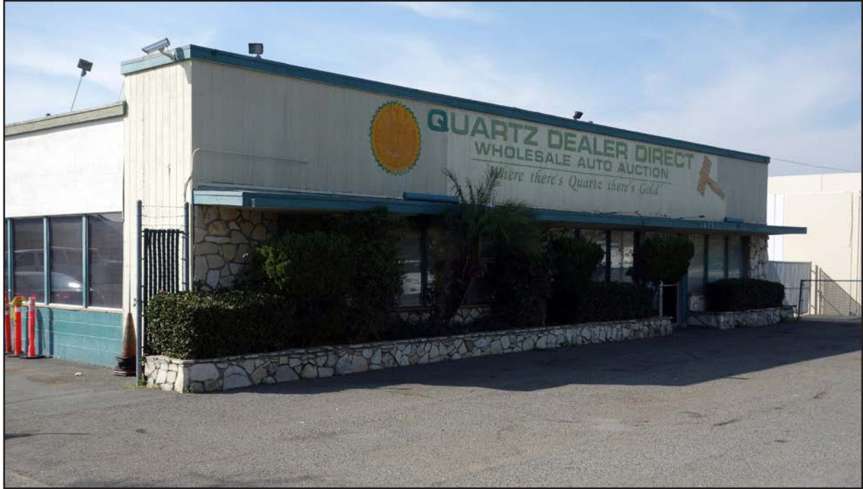
Photo 1. View looking northwest from the east part of the site showing the Quartz Auto Auction building at 633 South East Street.
