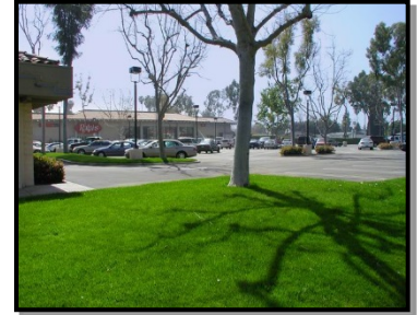
This commercial development, located at the southwest corner of Lincoln Avenue and Gilbert Street, provides an example of a Neighborhood Commercial center.
