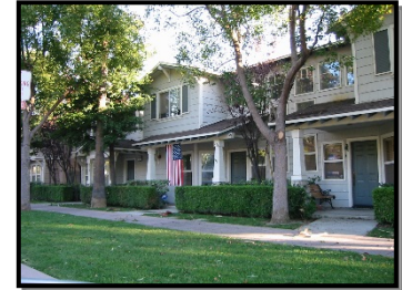
These townhomes in the Anaheim Colony are one example of the many varieties of residential types that can be built in the Low-Medium Density designation.
