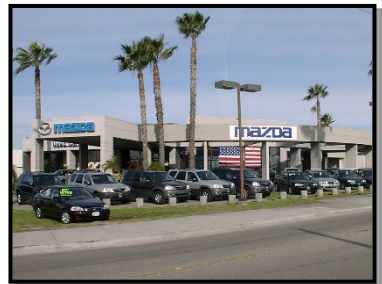
The General Commercial designation provides for a wide variety of commercial uses, including automobile sales.
