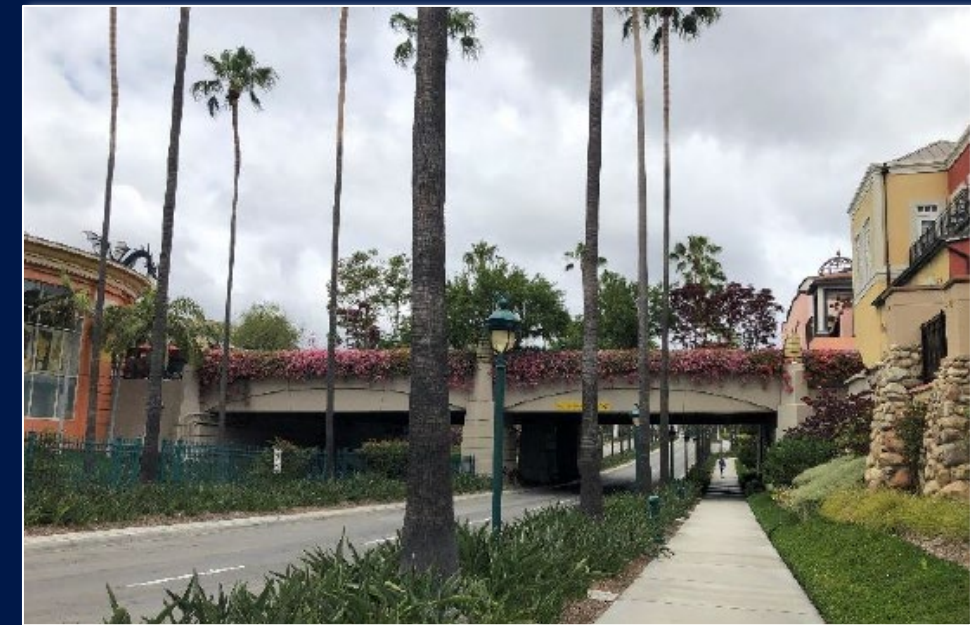
Existing Disneyland Drive Bridge
