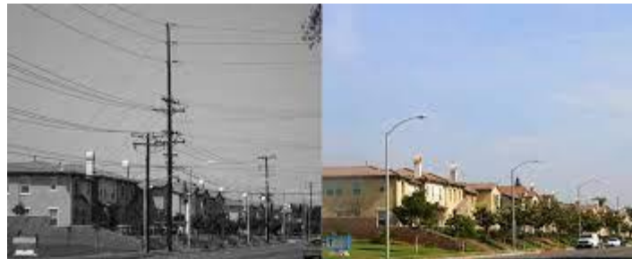
Example of Relocated Powerlines
