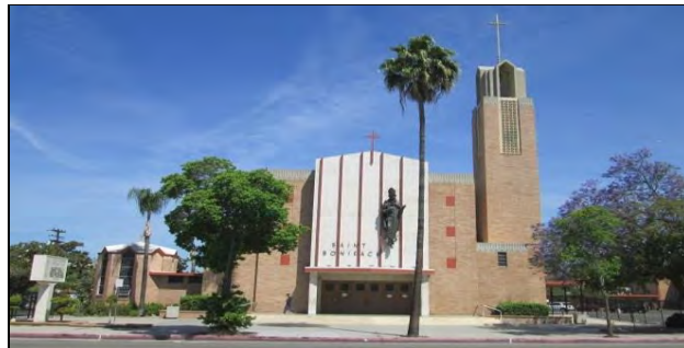
Façade, View to The North (April 20, 2016)
