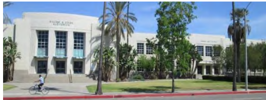
Façade (Partial), View to the North (April 20, 2016)
