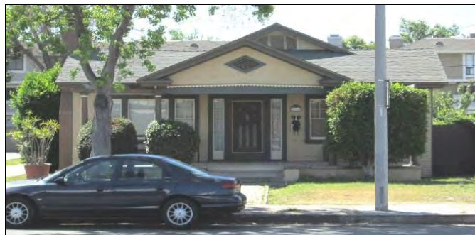
Façade, View to the South (April 20, 2016)
