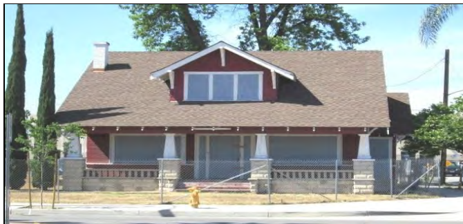
Façade, View to the North (April 20, 2016).
