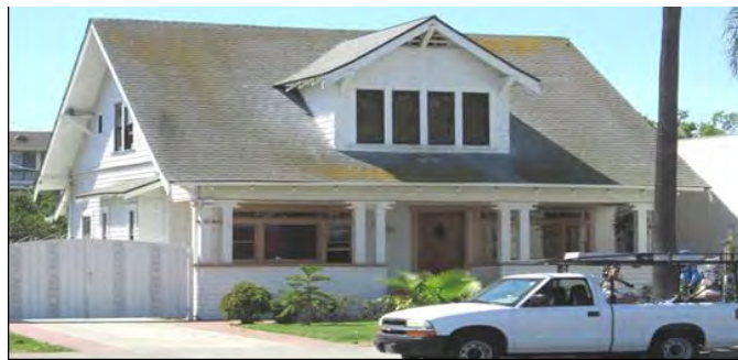
Façade and East Elevation, View to the Southeast (April 20, 2016)
