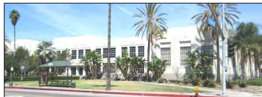
Façade (Partial), View to the North (April 20, 2016)
