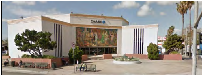
Façade and east elevation, view to the west (Source: Google April 2015).
