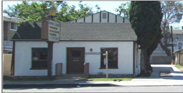
Façade, View to the South (April 20, 2016)
