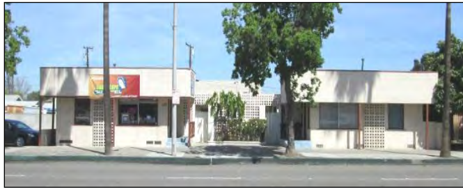
Façade, View to the North (April 20, 2016)
